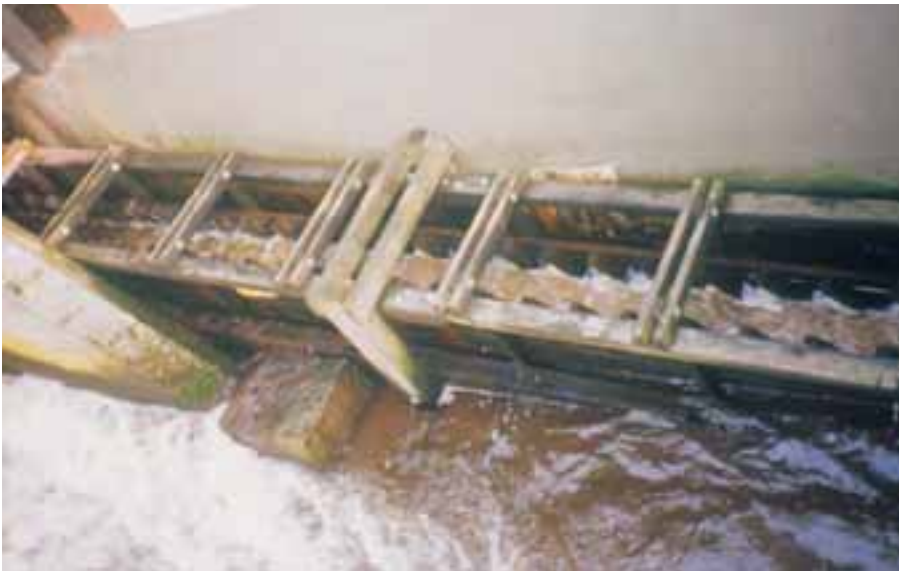
Figure 5.30: Denil pass made of wood Gifhorn/Ise (Lower Saxony)
