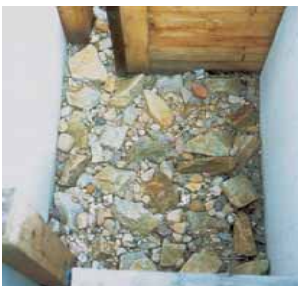
Fig. 3.14: Coarse bottom substrate in a slot pass; Lower Puhlstrom weir in the Unterspreewald (Brandenburg)
