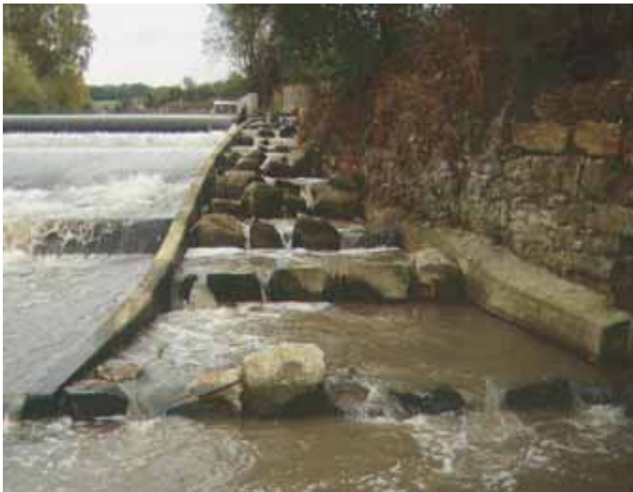
Figure 4.37: Uhingen/Fils rough-channel pool pass
