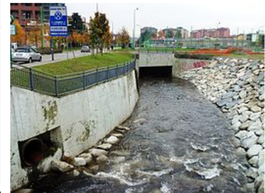
Tunnelling of Seveso River
